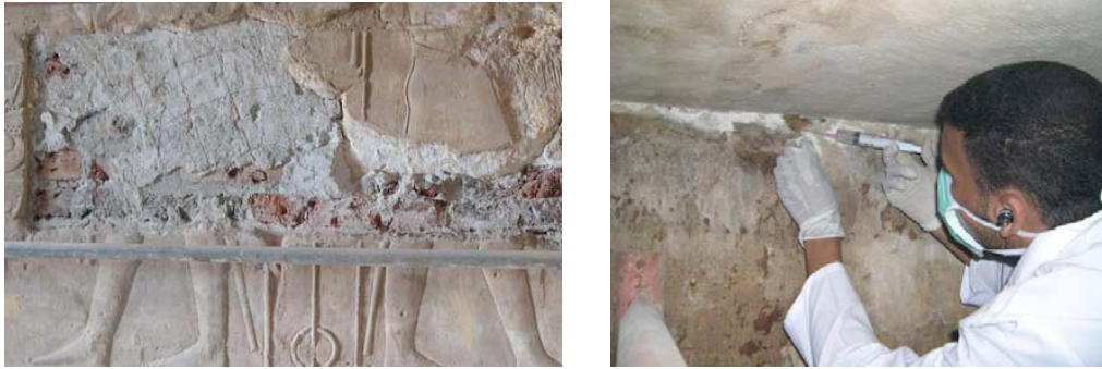
Removal of cement mortars, and consolidation of altered sandstone support © A. Asperti.
