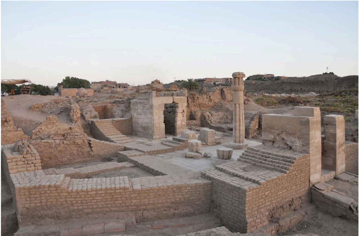
The chapel of Osiris Wennefer Neb Djefau after restoration of the mudbrick walls, the pavement and the naos © L. Coulon.
