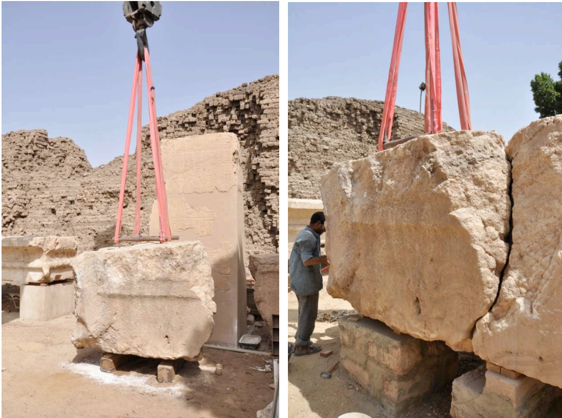
Fragment n° 1 lifted by the crane and approached close to the main fragment © Cnrs-Cfeetk/A. Garric.
