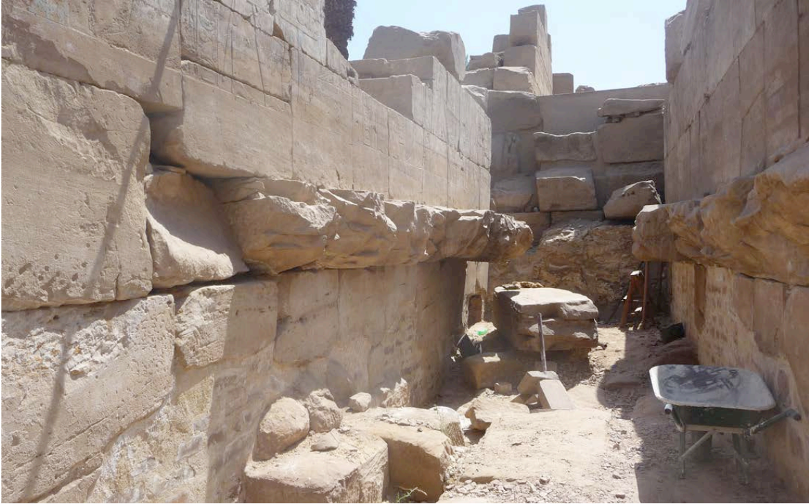
General view of the northern storeroom 7 during the work © Cnrs-Cfeetk/Chr. Thiers.
