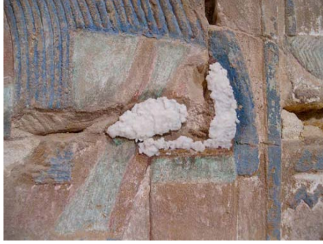
Cellulose powder compress applied to treat a darkening of polychromy, and detail of the painted reliefs before cleaning © A. Asperti.
