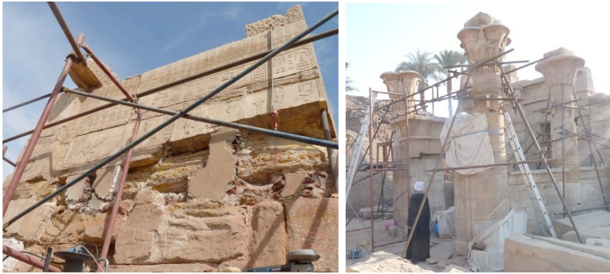
Gates B and E: Removal of plaster and brick/cement fillings, supporting and consolidation with ethyl silicate © Cnrs-Cfeetk/L. Pieri.
