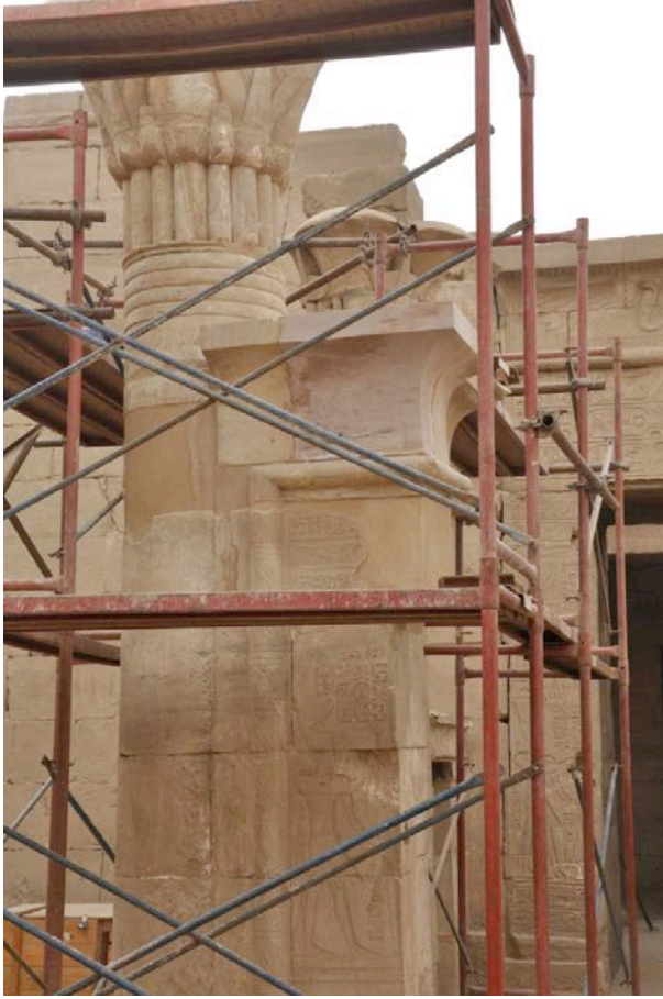
New cornice block at the top of the Gate E. © Cnrs-Cfeetk/A. Garric.
