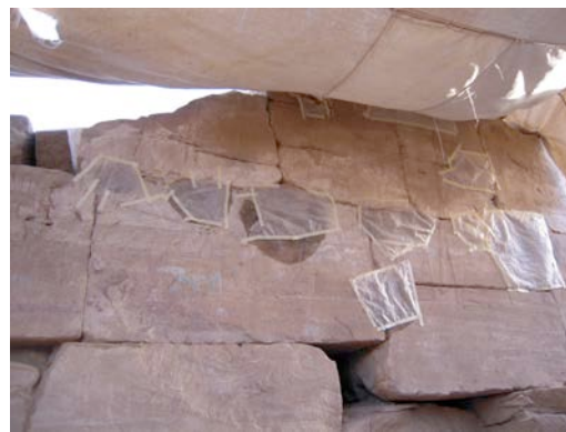
A cleaning and a pre-consolidation of the painting were made in order to silicate the damaged stones © Cnrs-Cfeetk/C. Bourse.
