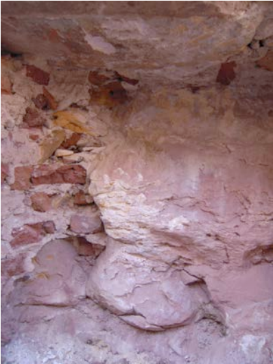
The old cement and brick masonry
