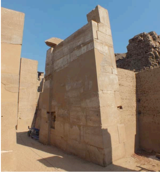
Gate B and E: After consolidation treatment, new fillings and plasters made of sandstone and lime mortar © Cnrs-Cfeetk/L. Pieri.
