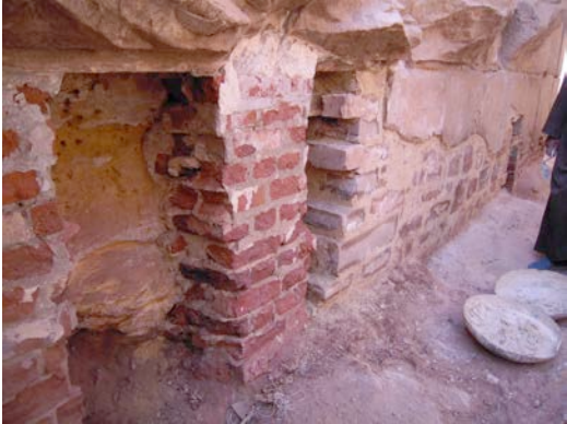
The new lime and stone masonry © Cnrs-Cfeetk/C. Bourse.
