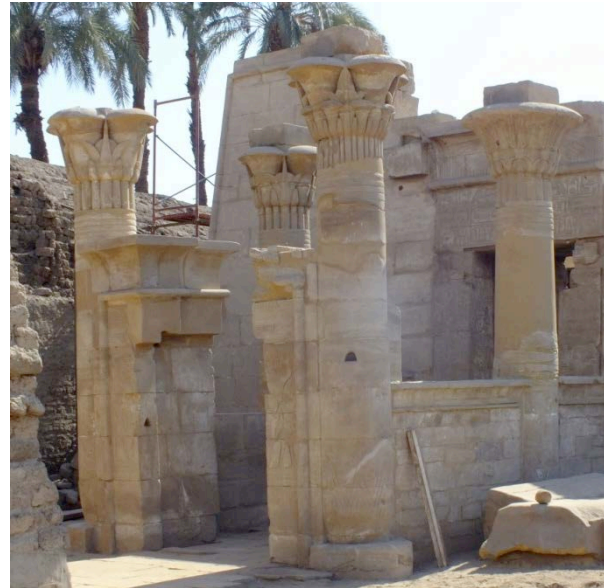
Gate B and E: After consolidation treatment, new fillings and plasters made of sandstone and lime mortar © Cnrs-Cfeetk/L. Pieri.
