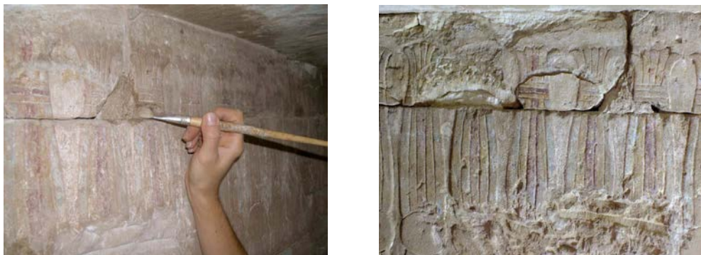
Consolidation of original coatings, and bonding of a detached sandstone fragment © A. Asperti.
