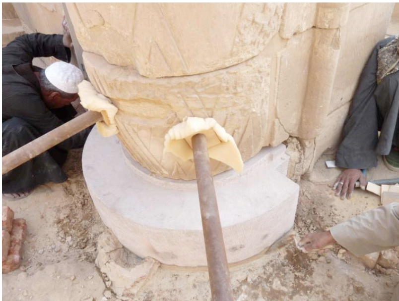
New column base on Gate E © Cnrs-Cfeetk/A. Garric.
