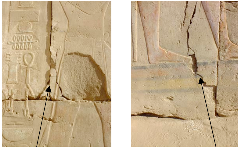
These pieces had to be fixed. To the left, we used Araldite 2015 because we could remove it. To the right, we made infiltrations © Cnrs-Cfeetk/C. Bourse.
