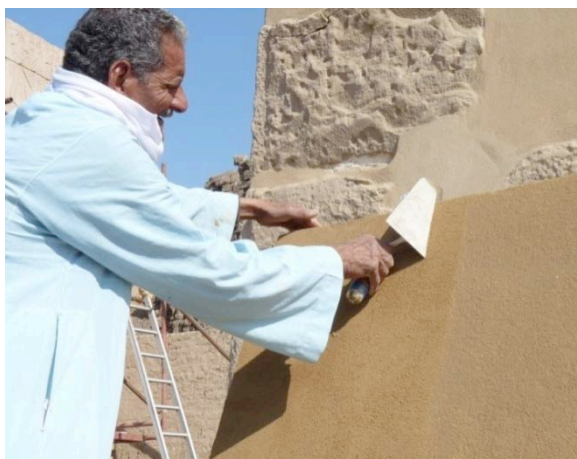
Colored finish plaster: Left powdery finish with trowel; Right, close finish with dry sponge.
