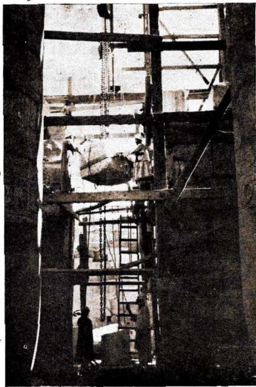
(b)—Raising a block by crane in order to replace it in its original position.
