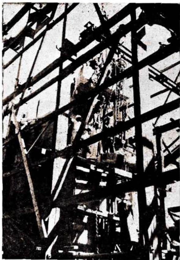
(c)—Workmen using the crane for lifting blocks to the top of the Wall.
