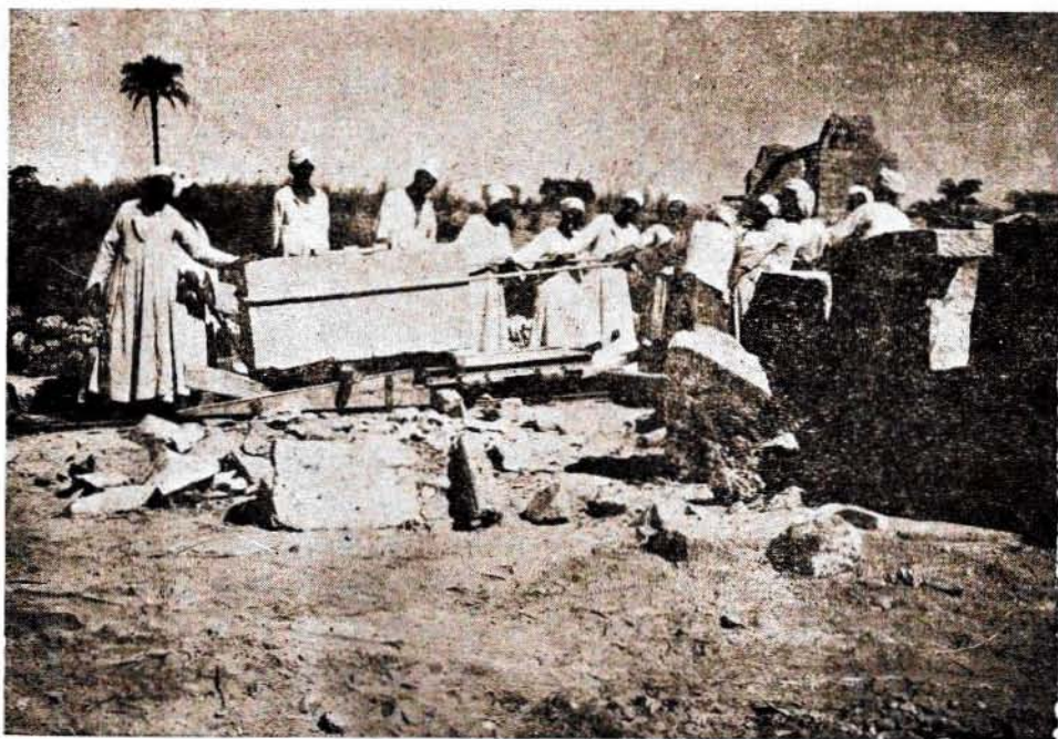
(d) Block dragged on rollers and decauville-car in order to be replaced in its original position.
