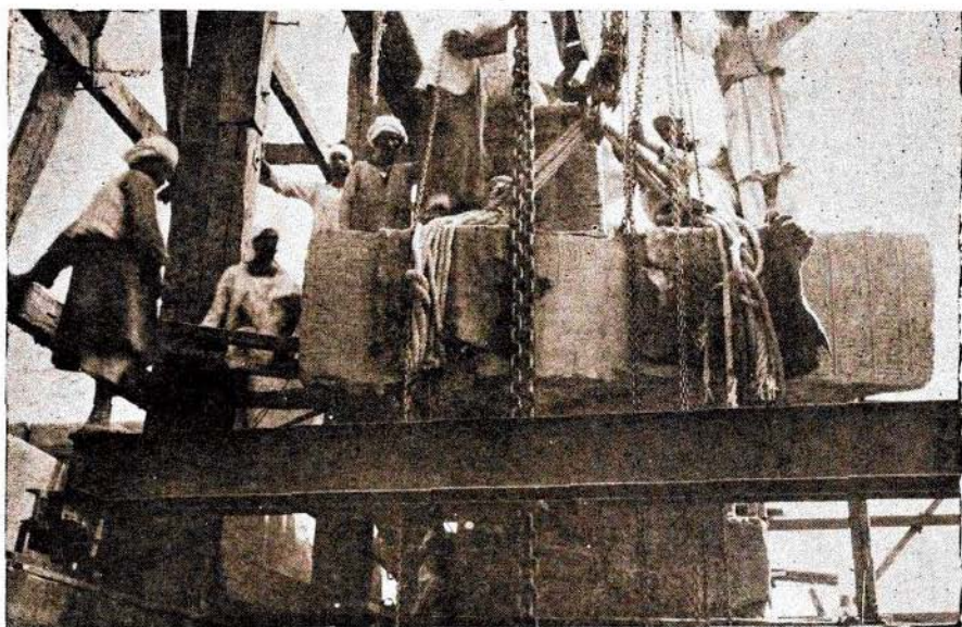
(a)—Raising a large block tied with rope on pad by means of tackle-and-block.
