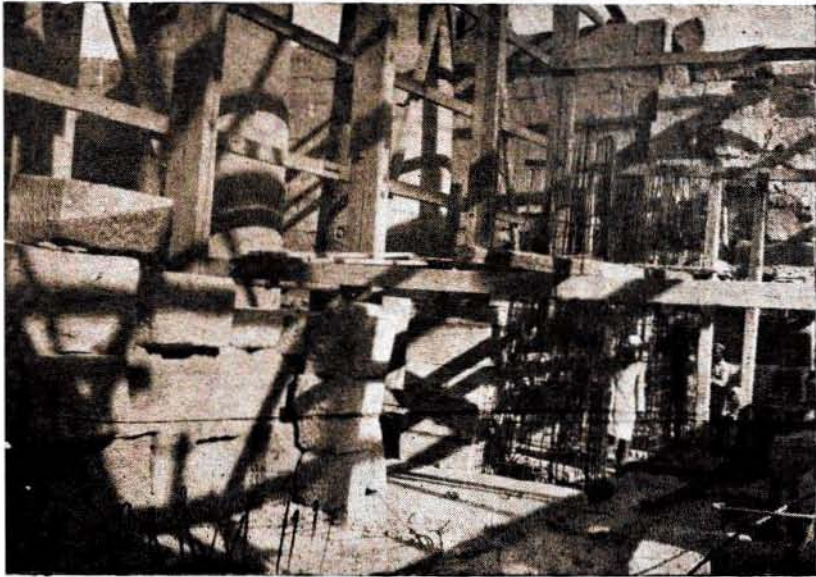
First stage of building concrete abutments.
