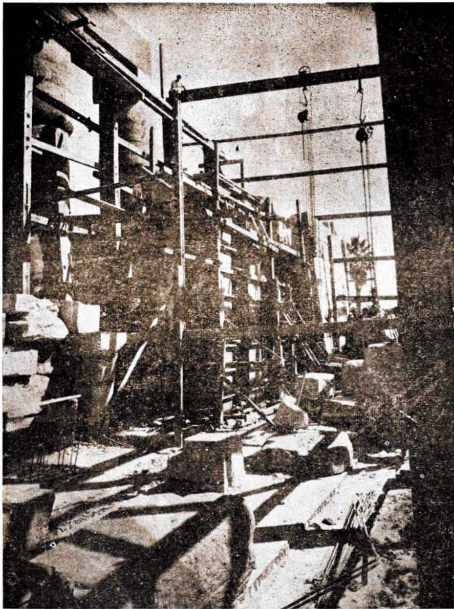
Back of Wall supported by concrete abutments and preparation for reconstruction of Pylon on concrete foundation.
