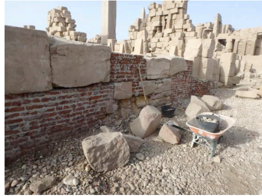
Only the colored coating has been removed, showing a cement and bricks masonry. © CNRS-CFEETK/C. Bourse.
