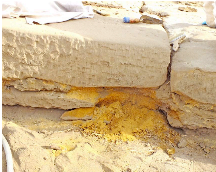
Arenised sandstone during its purge. © CNRS-CFEETK/C. de Oliveira.
