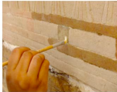
East wall: Consolidation of the pigments Klucel G at 3%. © CNRS-CFEETK/M. Lefevre.
