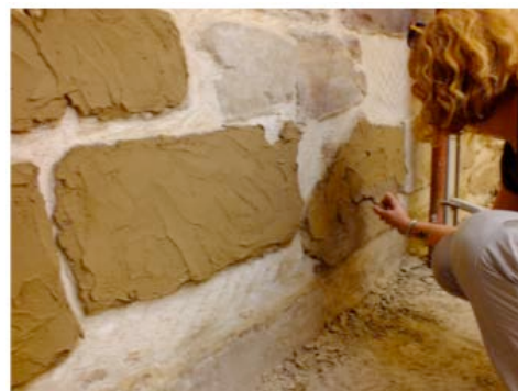
South wall: Removing salt with hiba (Egyptian clay). © CNRS-CFEETK/M. Lefevre.
