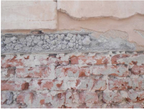
Only the colored coating has been removed, showing a cement and bricks masonry. © CNRS-CFEETK/C. Bourse.
