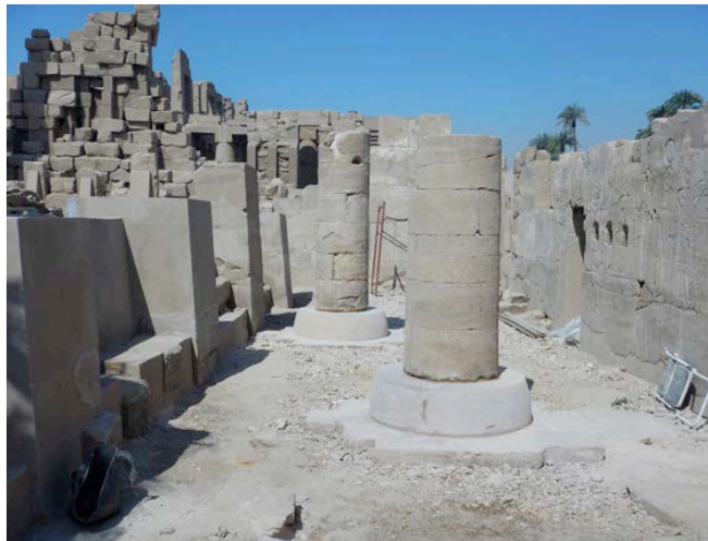
The two columns standing upon their new bases. © CNRS-CFEETK/Chr. Thiers.
