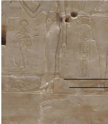
Filling in lime and sand mortar (1.3)
