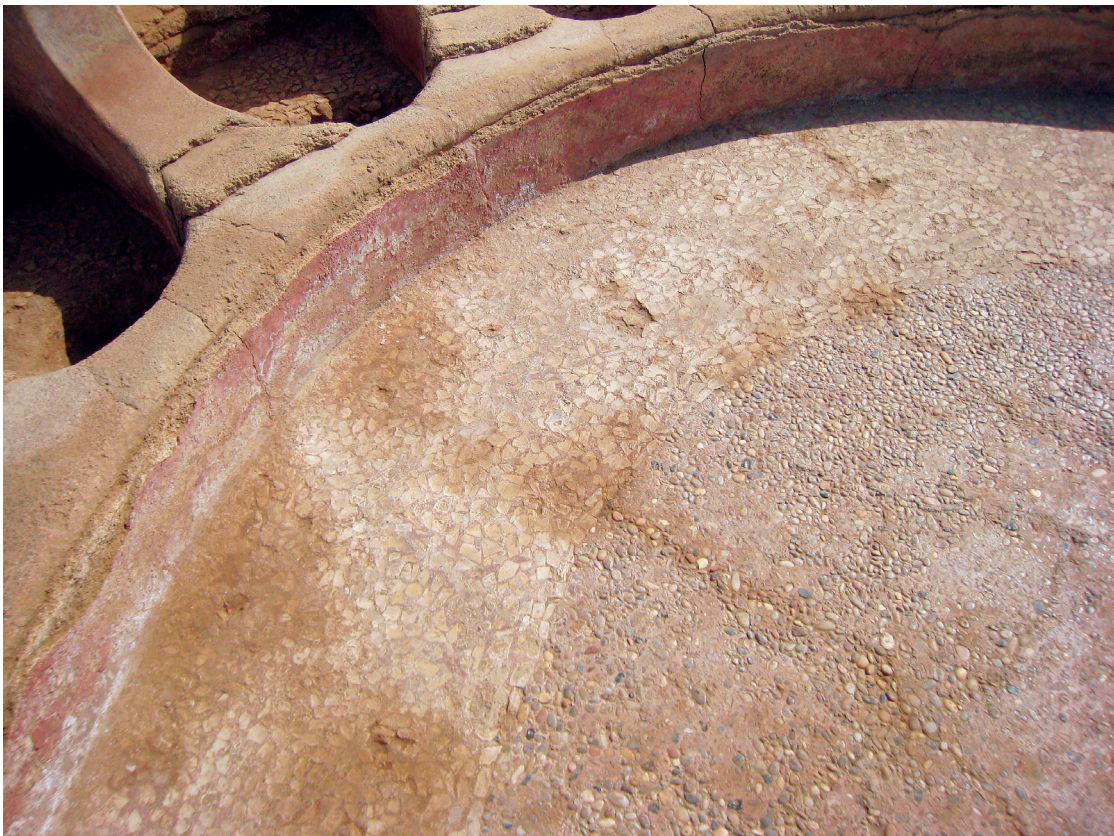
Fig. 21. Southern tholos , floor's detail © A.-M. Guimier-Sorbets.
