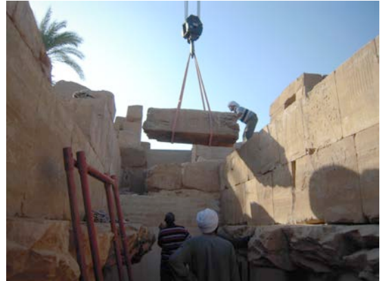
Holes were made before the block was replacing in order to fix the fiberglasses © Cnrs-Cfeetk/C. Bourse.
