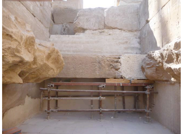
On its left side, flooring slab was fixed with three fiberglasses, and a coffering was made to its right side © Cnrs-Cfeetk/C. Bourse.
