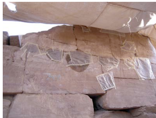
A cleaning and a pre-consolidation of the painting were made in order to silicate the sick stones © Cnrs-Cfeetk/C. Bourse.
