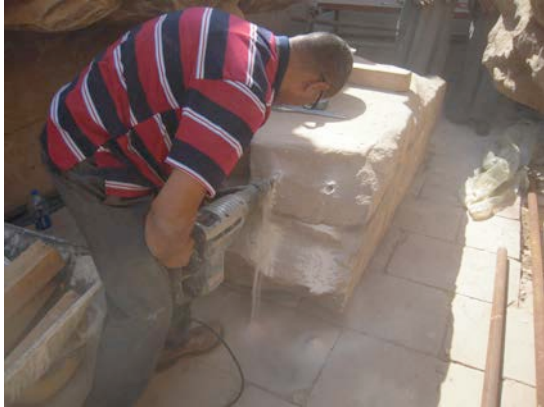
Holes were made before the block was replacing in order to fix the fiberglasses © Cnrs-Cfeetk/C. Bourse.
