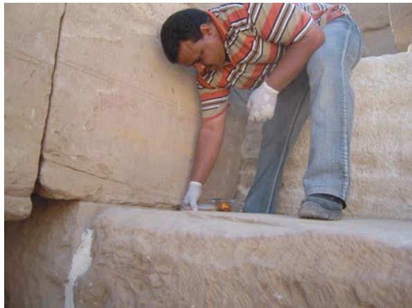
On its left side, flooring slab was fixed with three fiberglasses, and a coffering was made to its right side © Cnrs-Cfeetk/C. Bourse.
