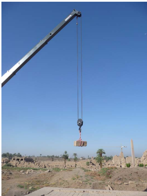
Ptolemaic block (2606) put back on the top of the northern wall of the courtyard.
