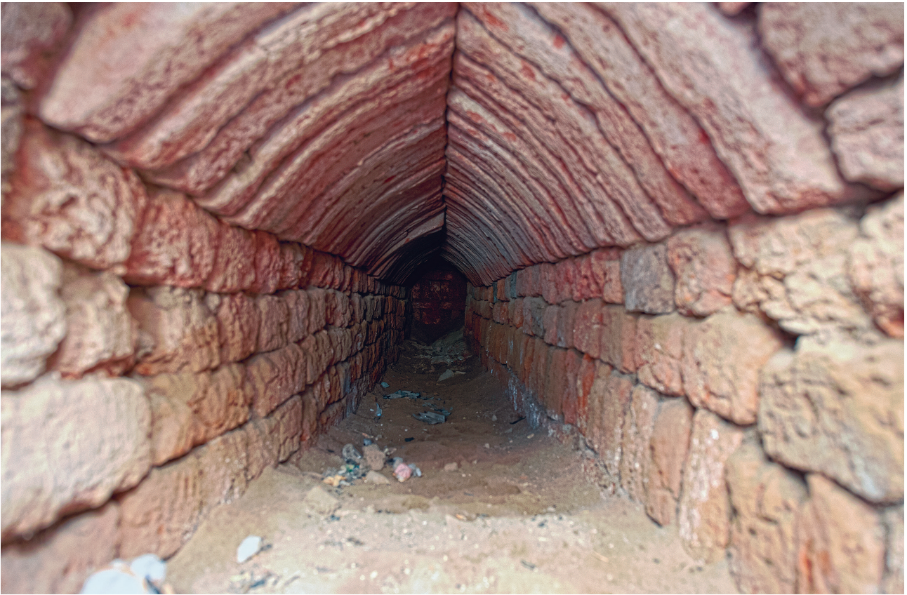
Fig. 12. The main drain of the wastewater system © O. Murray.
