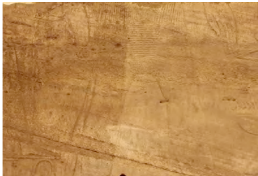
Mechanical cleaning (before at the left and after at the right). © CNRS-CFEETK/M. Lefèvre.
