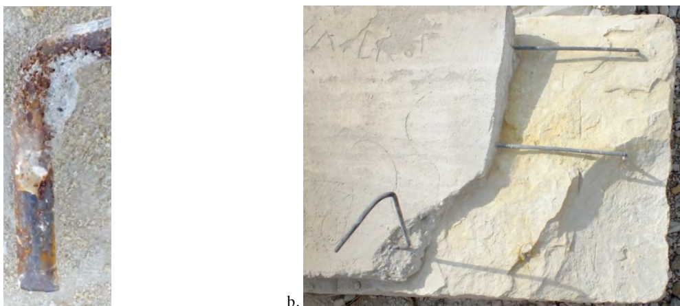
Oxidation state of a metal clip (a) and picture of one block during the withdrawal of the modern restorations (b). © CNRS-CFEETK/L. Antoine.
