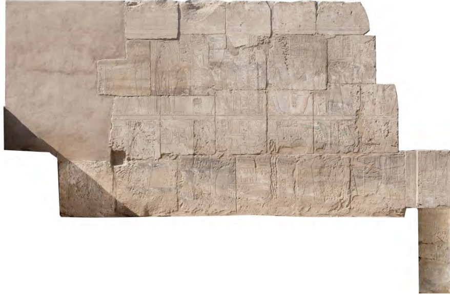
Orthophotograph after photogrammetric treatment of the South wall in the "Sokarian room" 5. © CNRS-CFEETK/P. Mégard.
