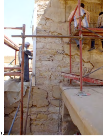
a. “Proto-crypt” on the south of the AKM.SK.4, after the first mortar (a). Upper area during the withdrawal of the cement (b). © CNRS-CFEETK/L. Antoine.
