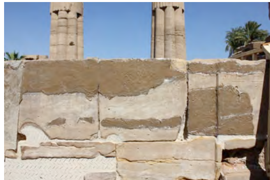
Desalination with compress of hiba -Attapulgate (north wall of AKM.SX.3). © CNRS-CFEETK/M. Lefèvre.
