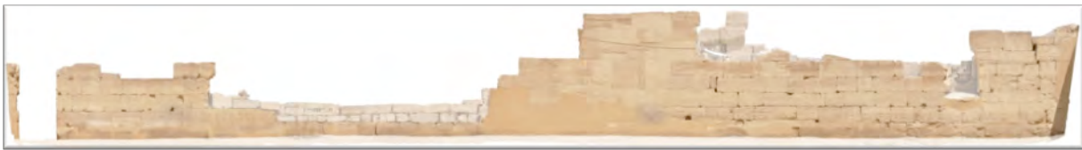
Orthophotograph of the west side of the East Wall. © CNRS-CFEETK/A. Garric.
