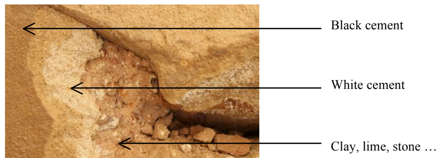
Different coats of the restoration’s mortar. © CNRS-CFEETK/M. Lefèvre.
