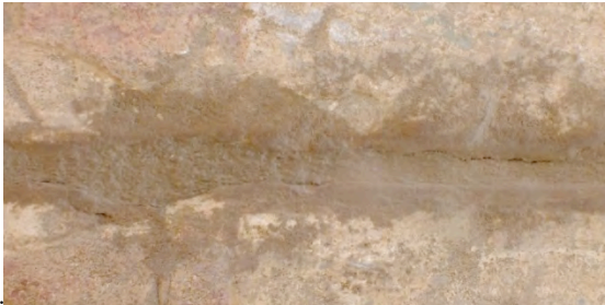
Localized loss of adhesion of the make layer (a), ongoing consolidation by PLM injection (b). Modern mortar overflowing on the stone and the painting (c), test of mechanical cleaning (d). © CNRS-CFEETK/L. Antoine.
