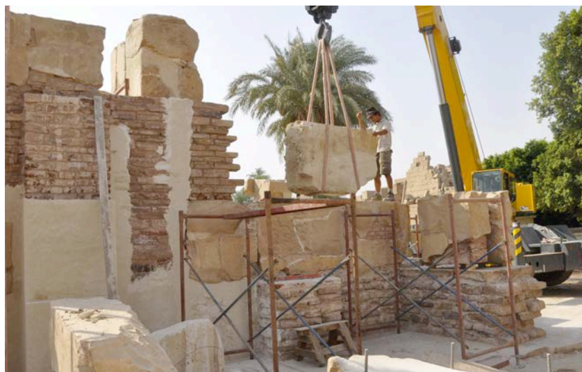
Block of the wall 1 being laid © Cnrs-Cfeetk/A. Garric.
