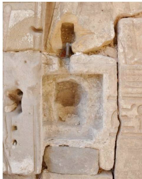
Locking system of the Gate B, before and after the removing of the mortar © Cnrs-Cfeetk/O. Bergès.
