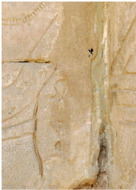
Detail of old mortar covering the relief © Cnr-Cfeetk/O. Bergès.
