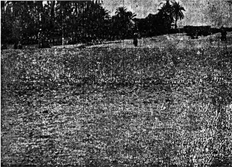
a. —The site before starting work, South side.
