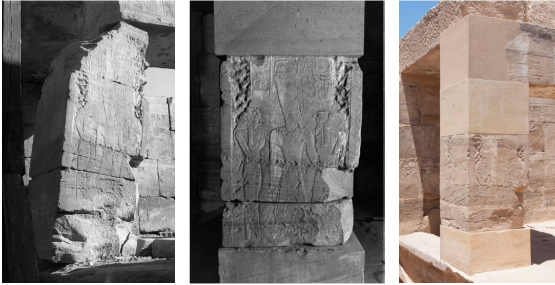
On the left, the pillar in 1967 ; in the middle in 1990 and on the right, the pillar after treatment. © CNRS-CFEETK 13/L. Antoine.
