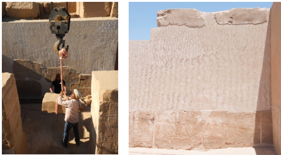
The move with the crane, and the two blocks on the east wall. © CNRS-CFEETK/L. Antoine.
