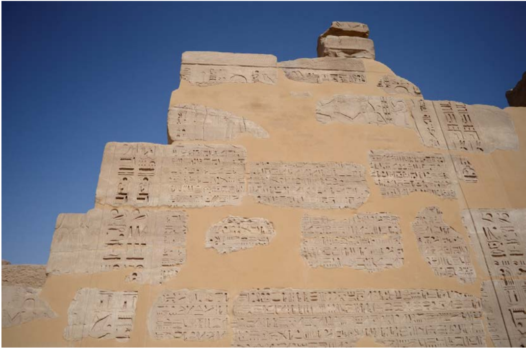
Reconstructed part of the west side of East wall. © CNRS-CFEETK/A. Garric.
