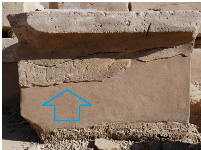
Traces of decoration under the cavetto of a pedestal in JB4. © A. Rickert, D. Mendel.
