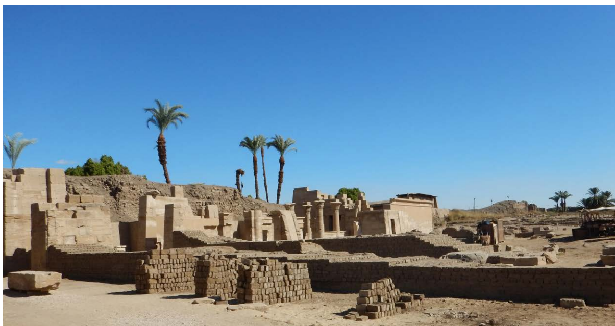
Final site management programme: reconstruction of mud bricks enclosure walls. © CNRS-CFEETK/Chr. Thiers.
