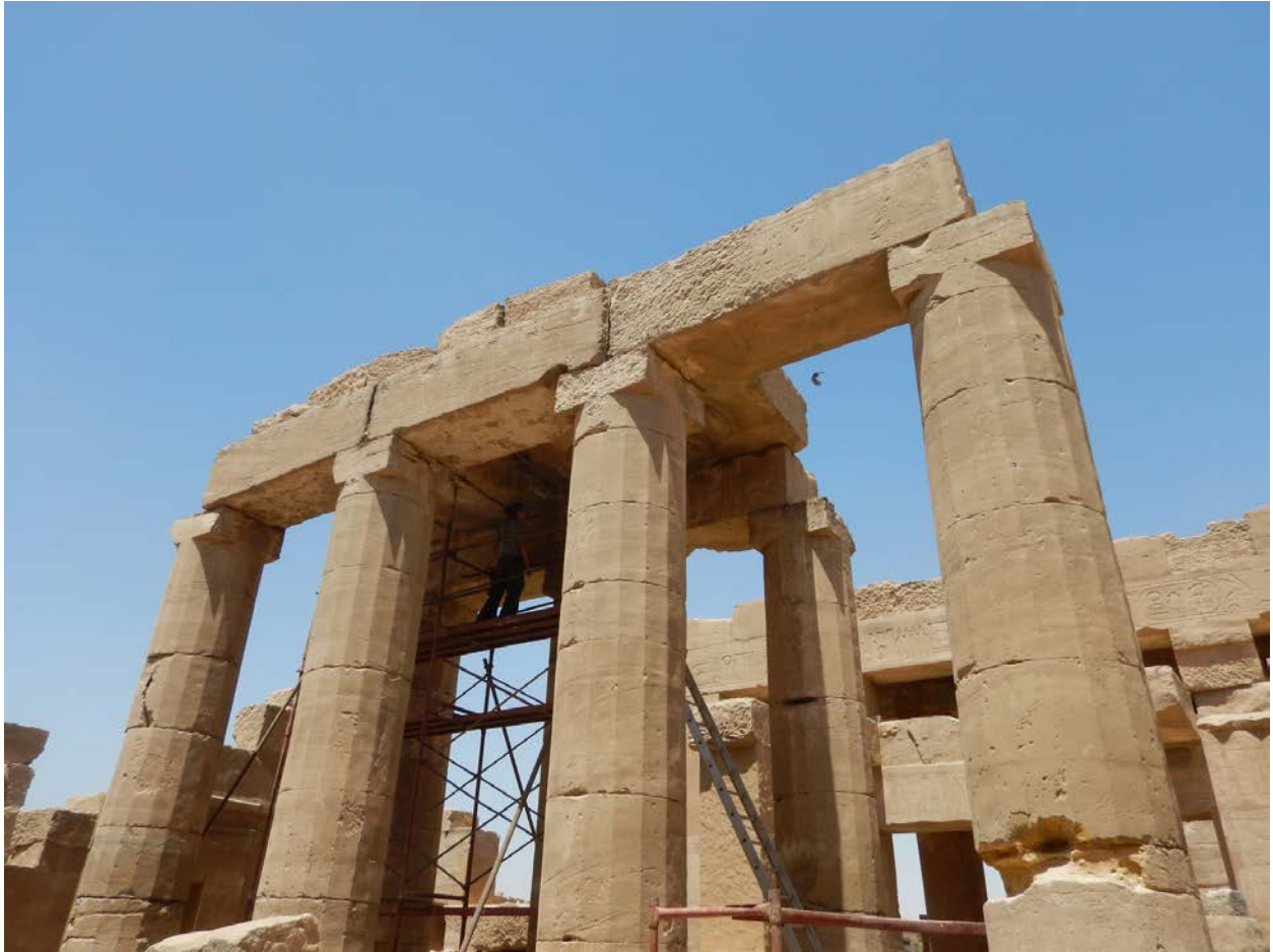
Conservation work on the hypostyle hall. © CNRS-CFEETK/Chr. Thiers.
