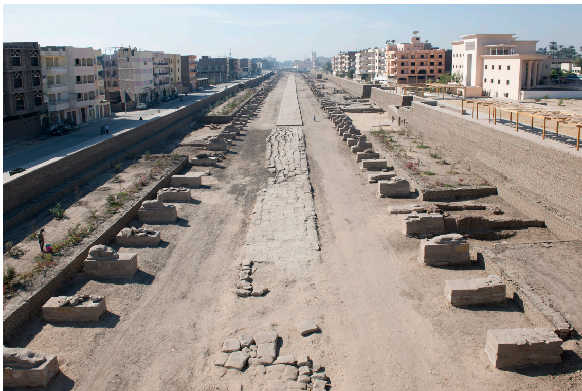
Fig. 11. The site behind the City library after restoration.
