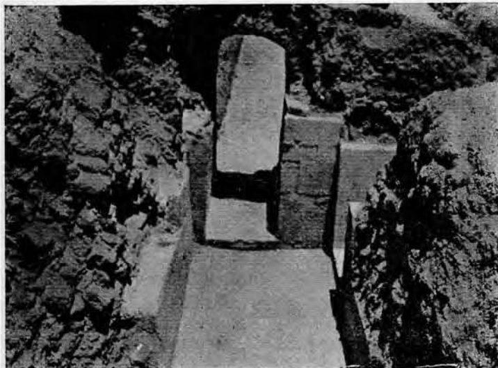
2. The brick walls lined with limestone blocks.
