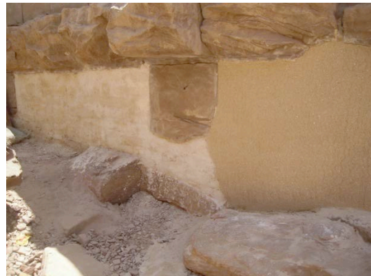
The new masonry with three layers of plaster: the first one, rich in lime whitewash (left photo) on which is placed the coated sided (right). Finally a colored coating covers the whole to fit better to the color of the stone © CNRS-CFEETK/C. Bourse.
