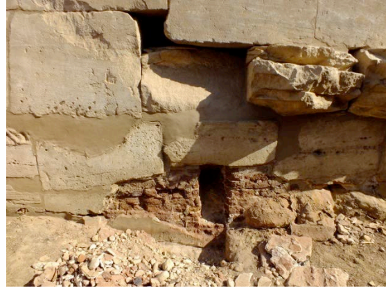
The shouks grew in the stone, breaking its molecular structure and strengthening the capillary rise (Photo of the outer corridor to the stores) © CNRS-CFEETK/C. Bourse.
