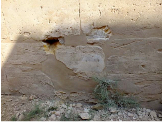
The shouks grew in the stone, breaking its molecular structure and strengthening the capillary rise (Photo of the outer corridor to the stores) © CNRS-CFEETK/C. Bourse.
