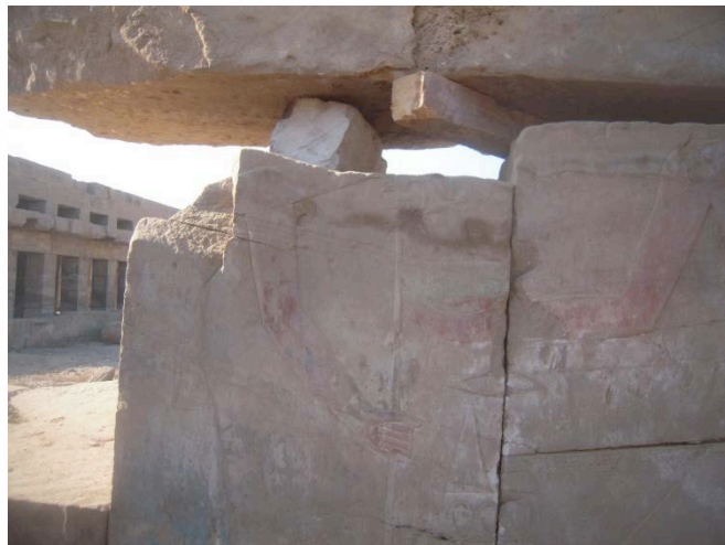
These photos taken in the MN5 show: left, a fractured block with a significant scaling and a gap at the bottom of the image. On the picture at the right, a brown moisture mark with salts is visible on the top block © CNRS-CFEETK/C. Bourse.
