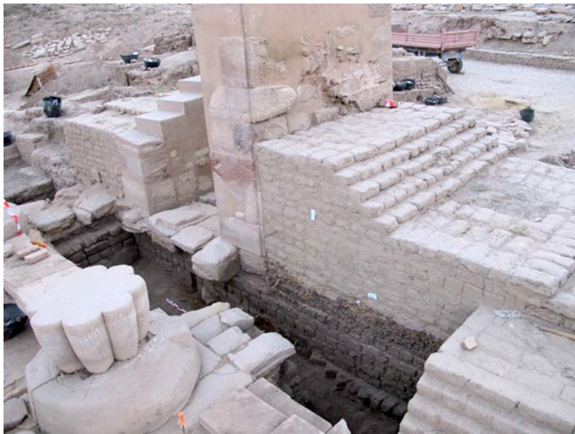
Mudbrick foundation of the southern part of the pylon and the first gate © Giorgi.
