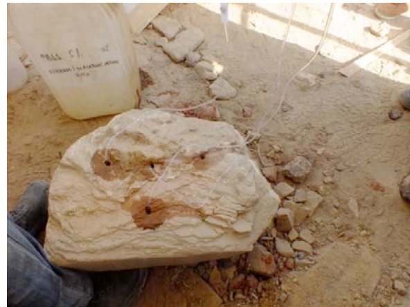
After having been pierced, the blocks are consolidated with ethyl silicate © CNRS-CFEETK/C. Bourse.
