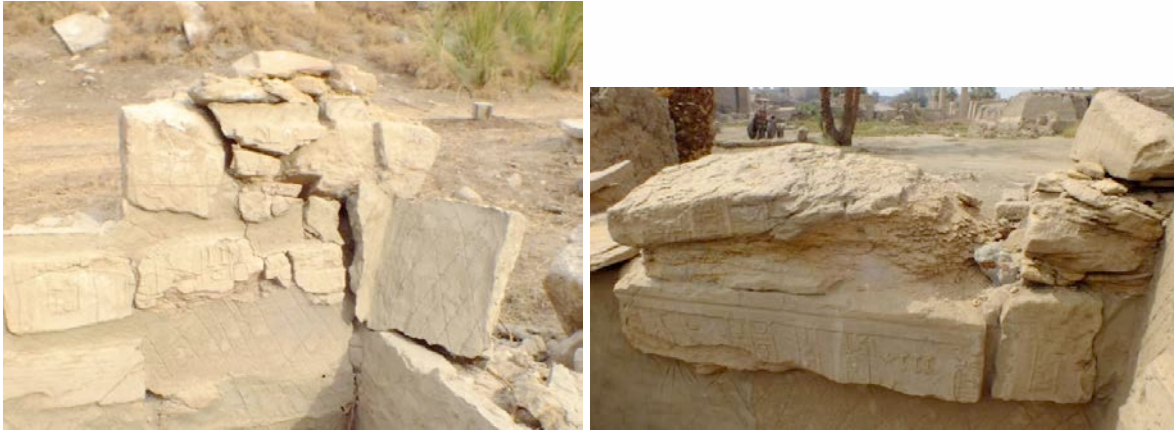
On the left picture, the block arenization is so advanced that it broke into fragments. The photo at right shows the state of the sandstone under the cement mortar © CNRS-CFEETK/C. Bourse.
