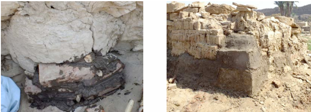
A new masonry, based on mud and reused red bricks, was established © CNRS-CFEETK/C. Bourse.
