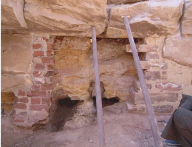
These photos were taken in the MN7. On the left picture, the ancient masonry made of cement and baked bricks is on the left while the new one made of stone and lime is visible to the right. The photo to the right shows the importance of the alteration of sandstone after withdrawal of the old masonry © CNRS-CFEETK/C. Bourse.
