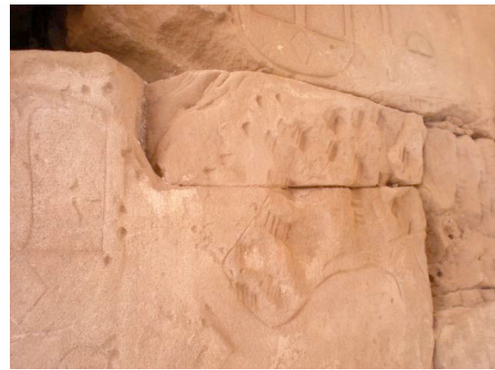
On the left picture, during the removal of the fragment, we discovered the original coating. The part in contact with the stone fragment was cleared in order to apply a new lime plaster (MN5) © CNRS-CFEETK/C. Bourse.
