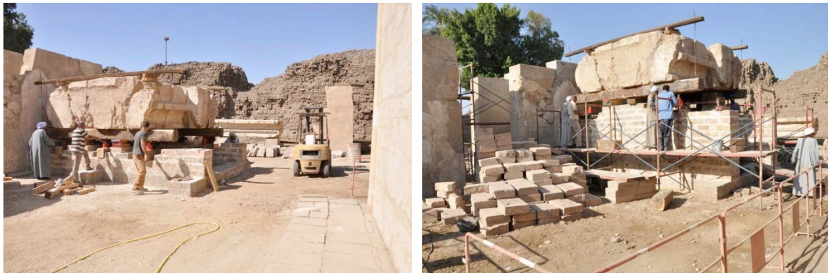
Manual lifting (with hydraulic jacks) of the ceiling stone © CNRS-CFEETK/A. Garric.
