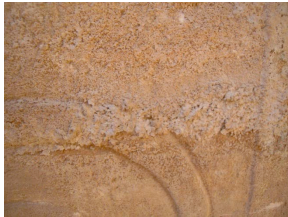
The left photo (MN7) shows cracked and raised polychromy. Over time, it may detach itself from the block. The right photo (MN7) reveals salts: with time, they were pushed and then mixed with the white preparatory layer. After several cycles of crystallization, they now make up this white granule layer © CNRS-CFEETK/C. Bourse.
