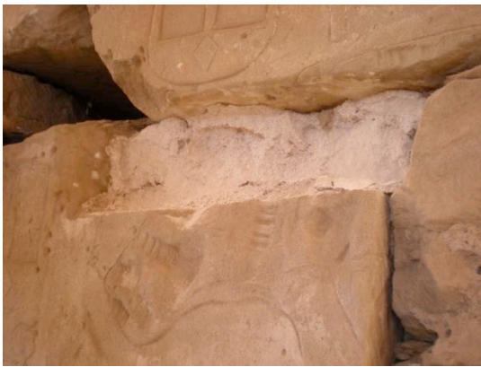
On the left picture, during the removal of the fragment, we discovered the original coating. The part in contact with the stone fragment was cleared in order to apply a new lime plaster (MN5) © CNRS-CFEETK/C. Bourse.
