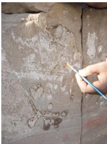
The original plasters were consolidated with ammonium oxalate in all stores (MN6) © CNRS-CFEETK/C. Bourse.
