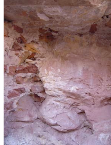
These photos were taken in the MN7. On the left picture, the ancient masonry made of cement and baked bricks is on the left while the new one made of stone and lime is visible to the right. The photo to the right shows the importance of the alteration of sandstone after withdrawal of the old masonry © CNRS-CFEETK/C. Bourse.
