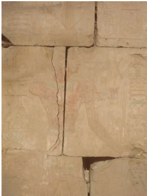
These photos taken in the MN5 show: left, a fractured block with a significant scaling and a gap at the bottom of the image. On the picture at the right, a brown moisture mark with salts is visible on the top block © CNRS-CFEETK/C. Bourse.
