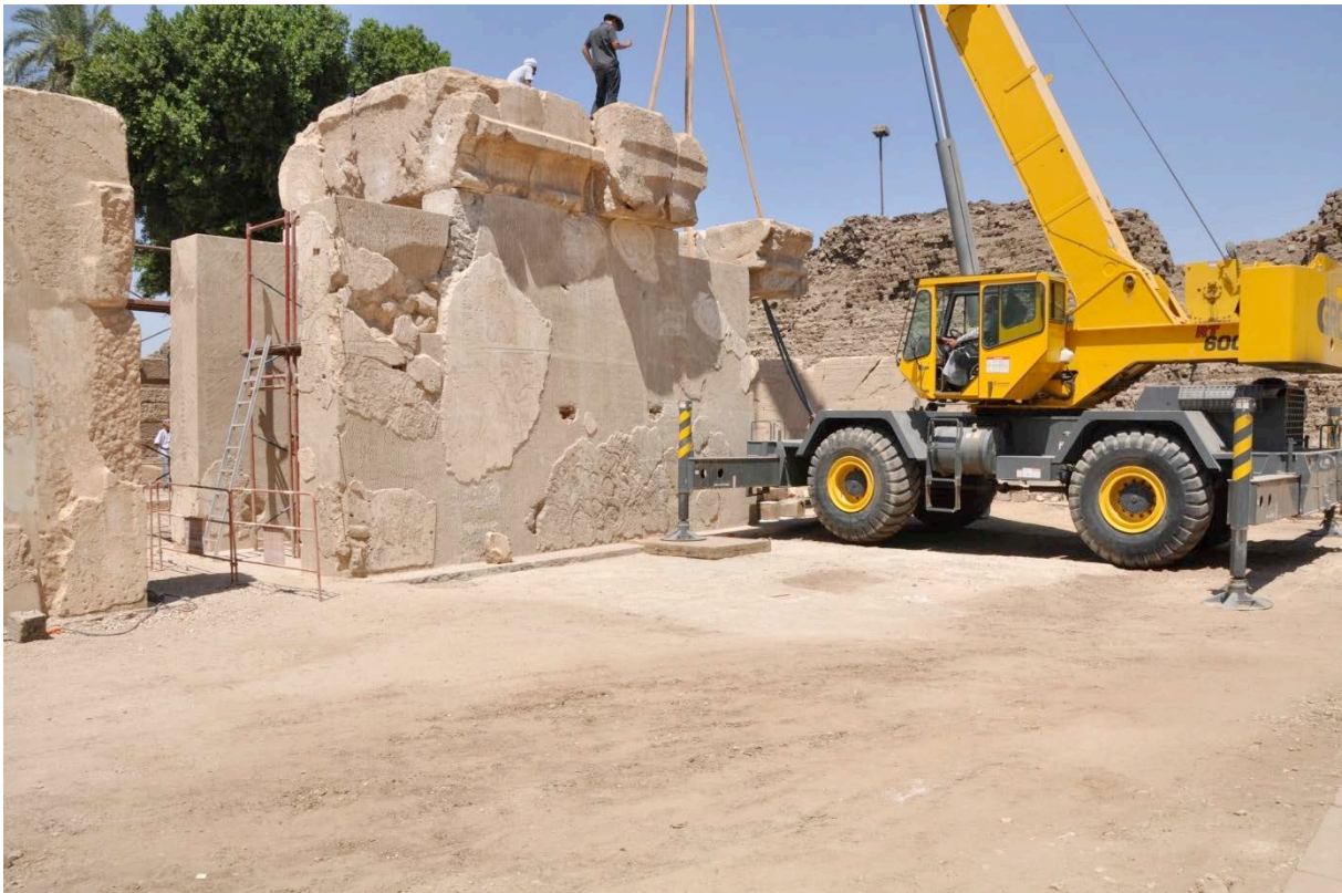
The lintel being lifted by the CFEETK crane © CNRS-CFEETK/A. Garric.
