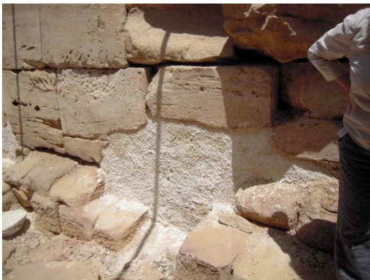
The new masonry with three layers of plaster: the first one, rich in lime whitewash (left photo) on which is placed the coated sided (right). Finally a colored coating covers the whole to fit better to the color of the stone © CNRS-CFEETK/C. Bourse.
